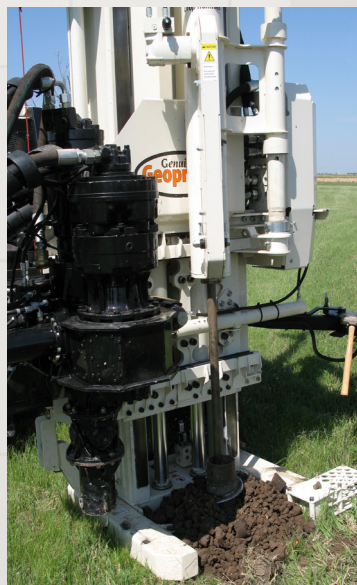
Auto Drop Hammer (Left) for geotechnical sampling
